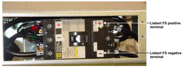
The Liebert FS cabinet is configured for top entry cables in standard configuration. The cables can also be run through the side panels. The Liebert FS cabinet does not accommodate bottom entry cables.
